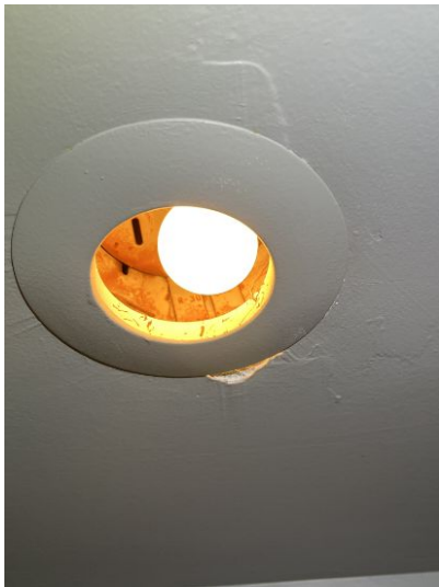
Bathroom - missing its protective cover
