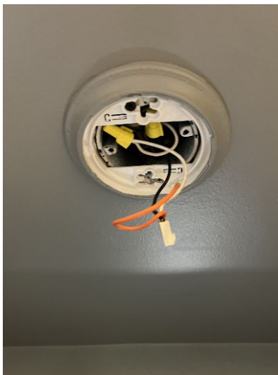
Bathroom - missing its protective cover
