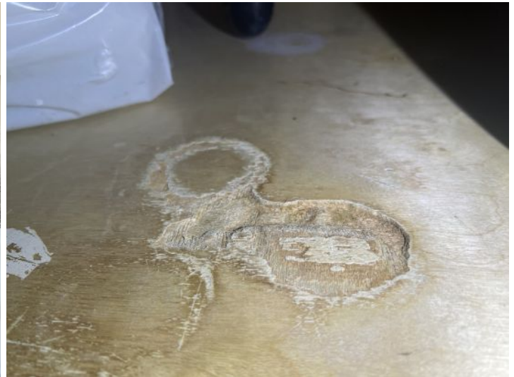
Moisture damage
