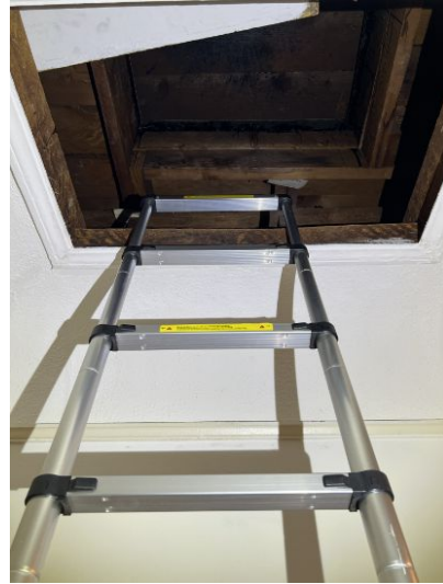
Access in unit 4
