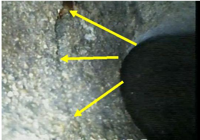
47' from access point
