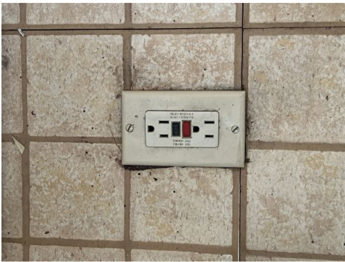
GFCI outlet located in the floor of the kitchen. This style of outlet is not meant to be in the floor. There is no protection to prevent outlet damage.
