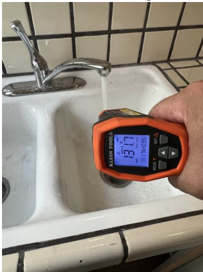
Unit 2 - Kitchen 131 deg F
