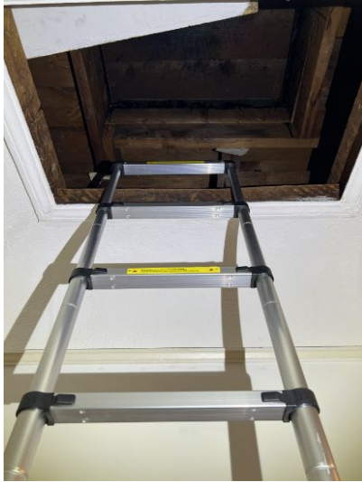
Access in unit 4
