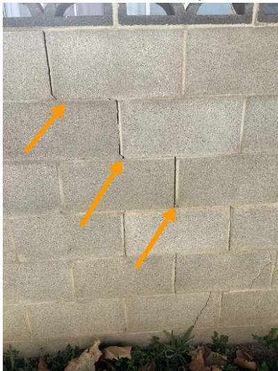
Step cracking
