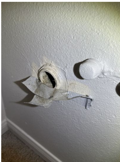
Closet of bedroom 1.
