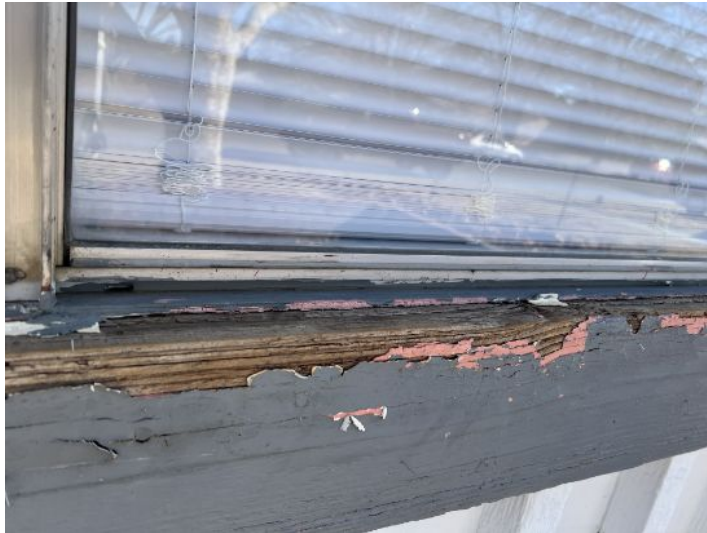
Exterior Exterior Trim Condition
