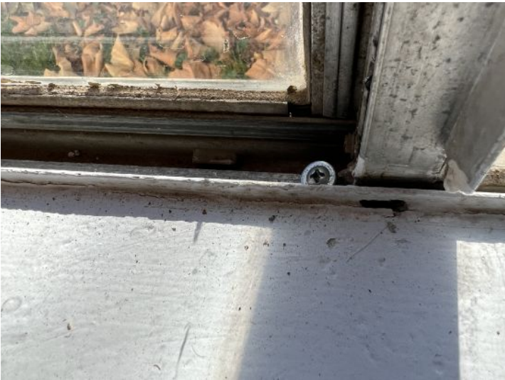
Screws being used as lock
