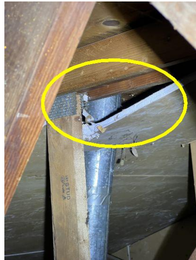
Firewall damage
