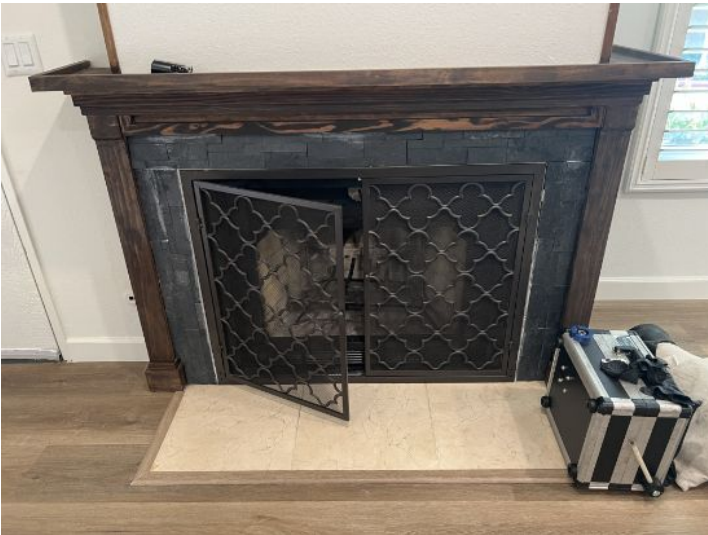
Under stairs - NOT GROUNDED PROPERLY
