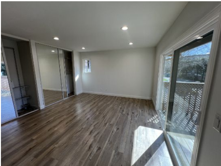
Bedroom 2 - NOT GROUNDED PROPERLY
