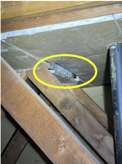
Firewall damage
