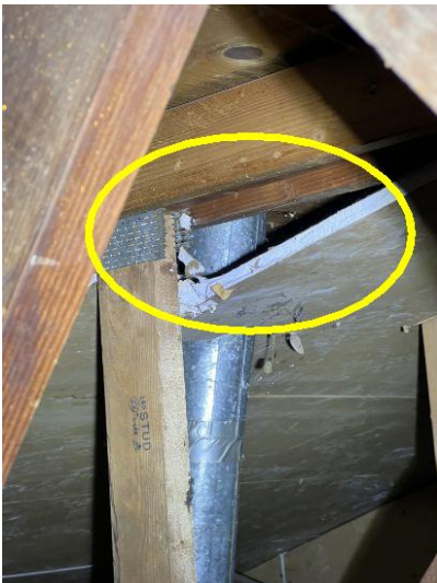
Firewall damage
